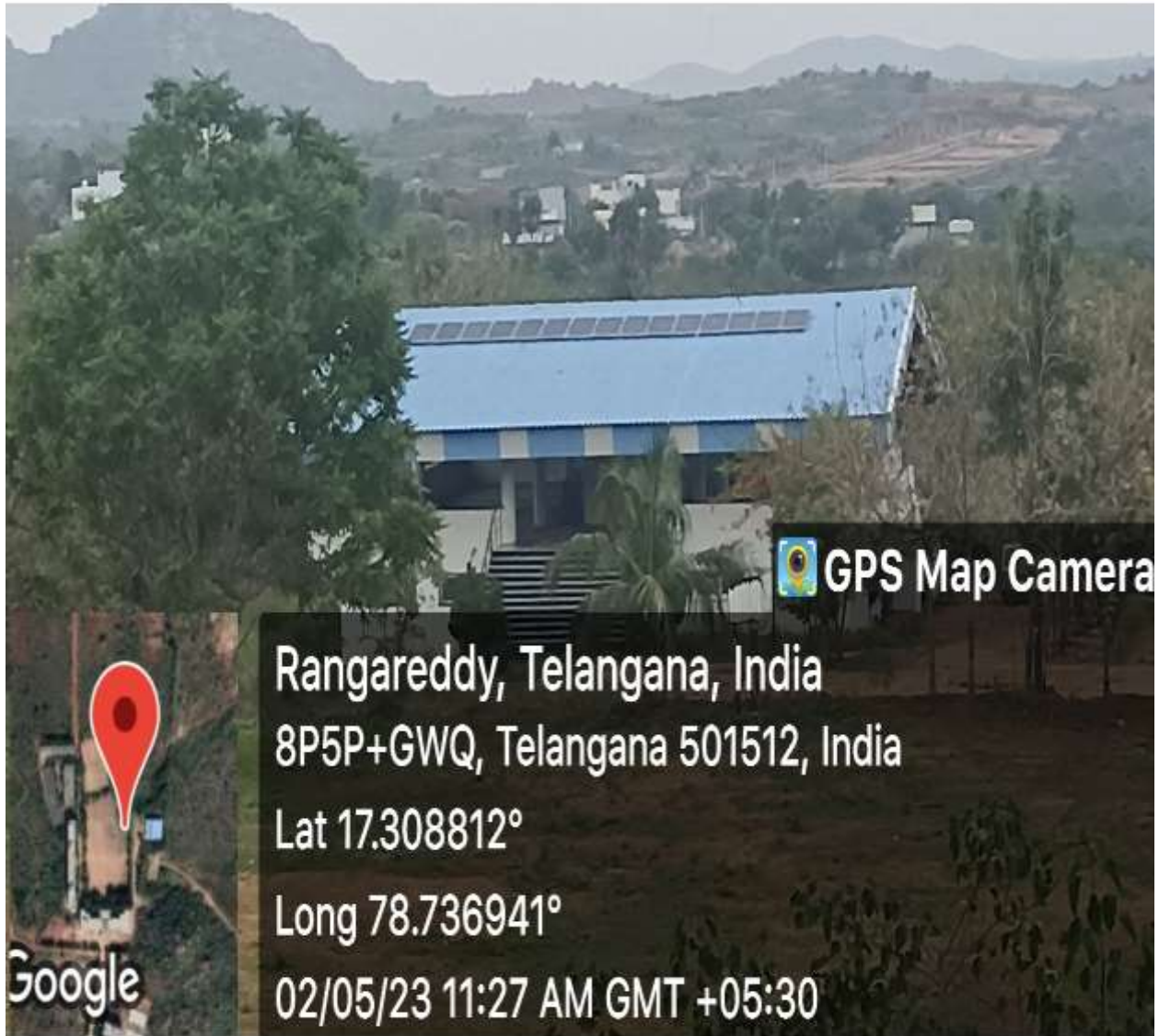
Front view of Solar Power plant with 5 KWp.
