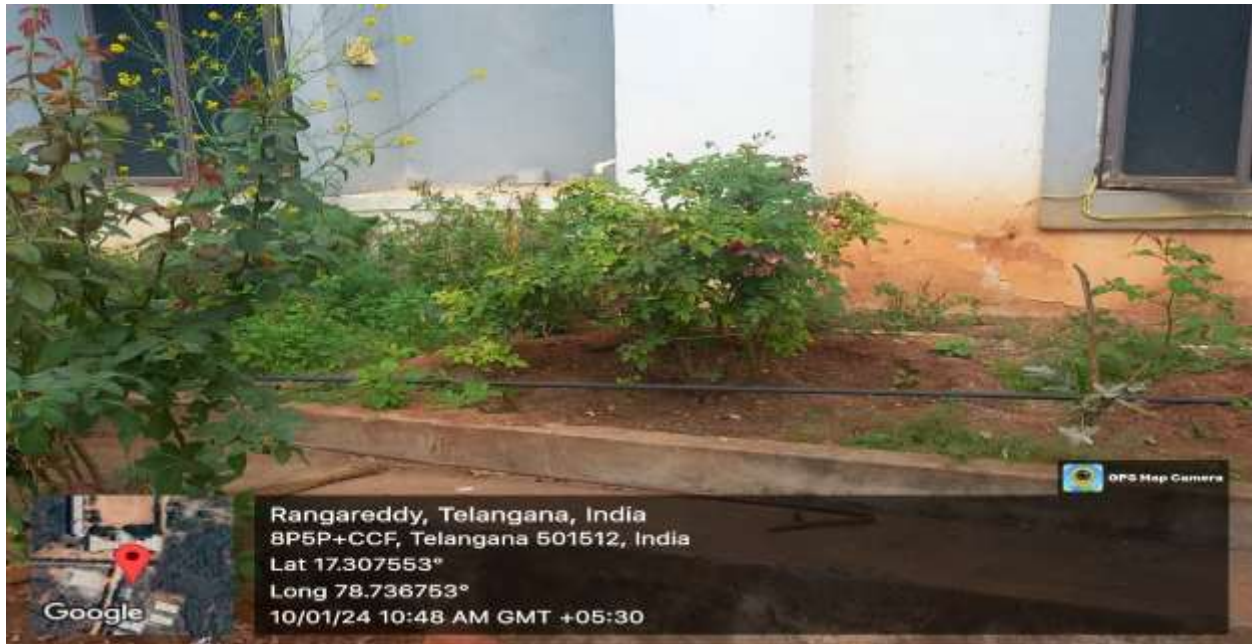
Sprinkle water system for plants in campus premises
