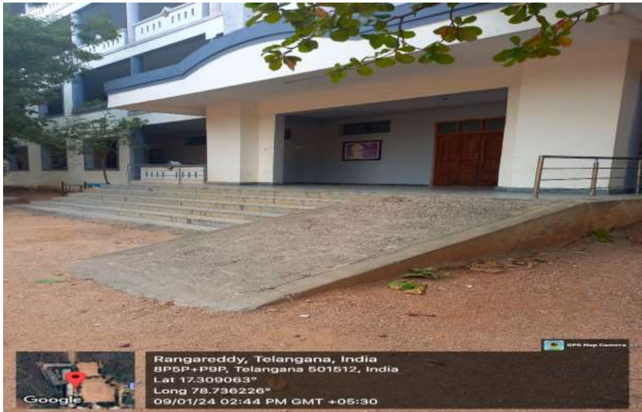
Ramp in B – Block
