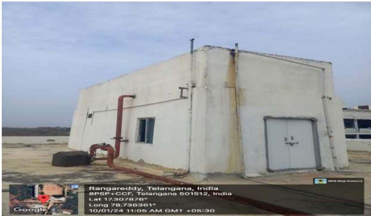
Overhead tank at AITH (A-Block)
