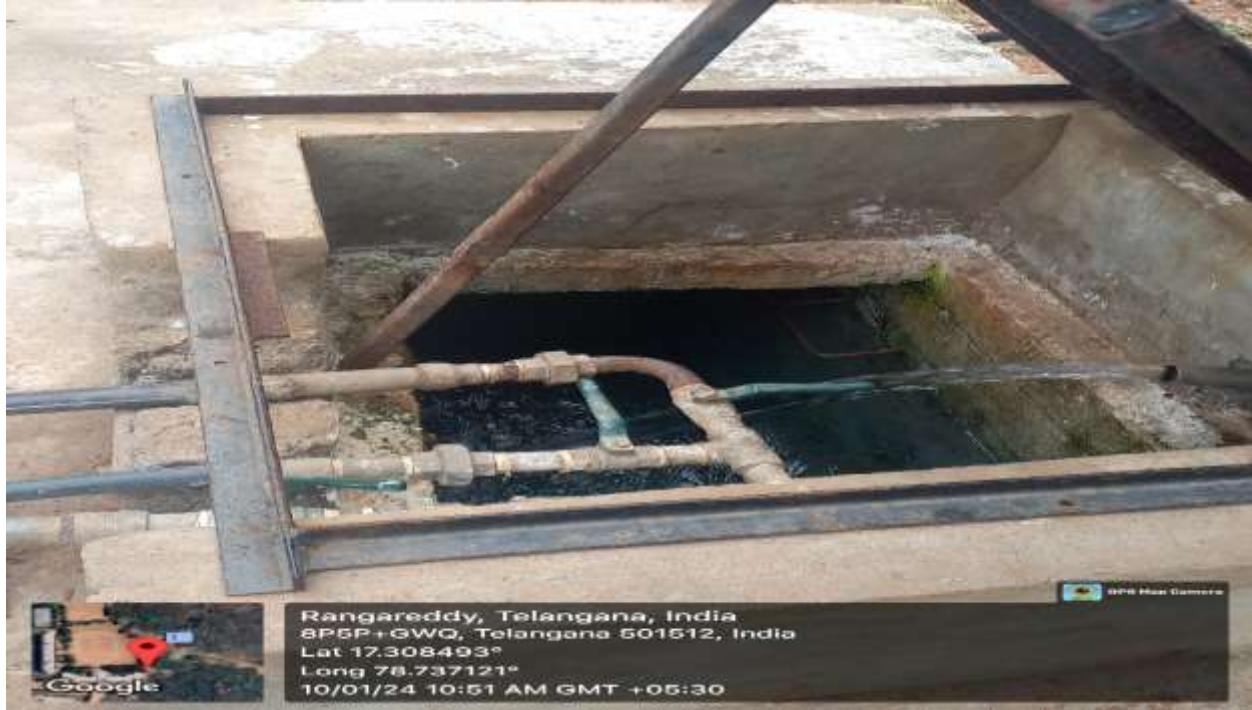
Construction of sump for storage of water at AITH
